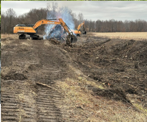
A series of drainage ditches like the one pictured left were closed to hydrologically restore the wetland at Farris.
