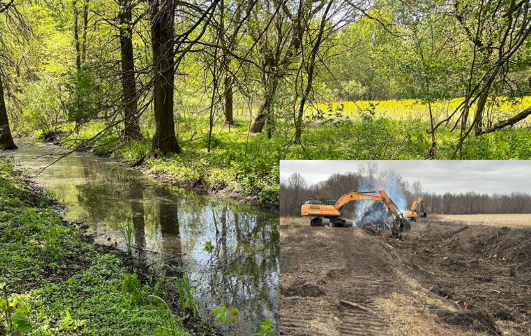
A series of drainage ditches like the one pictured left were closed to hydrologically restore the wetland at Farris.
